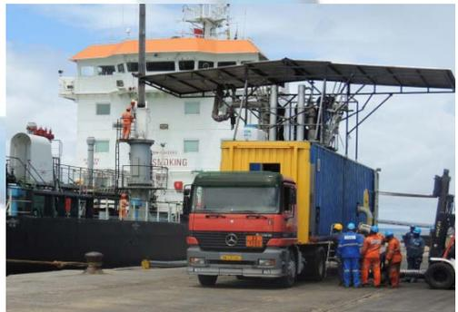
These units are an ideal solution for unloading a Bitumen carrier into containers for local storage and/or distribution. Flow rates of 160-200Mt/hr achievable, fitting well within Bulk Bitumen carriers normal allocated unloading time.
